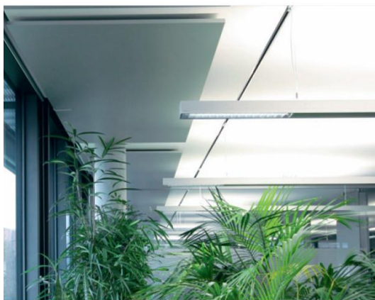
Velum as edge strip elements in combination with CCTC (installation next to the façade).
