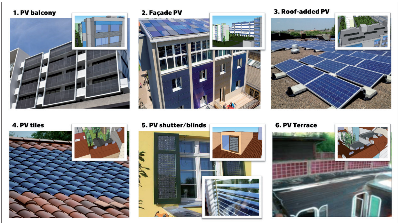
Fig. 3. Examples of architecturally integrated PV systems in the two building blocks: (1) PV balconies. Source: Etsprojects; (2) Coloured PV- facade. Source: Swissinso; (3) Roof-added PVs. Source: Cromwellsolar; (4) PV tiles. Source: Tradeford; (5) PV shutter and PV blinds. Source: COLT international, Solargaps; (6) PV terrace [26].
