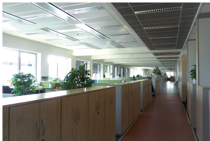
Obr. 1 Velkoprostorové kanceláře ve 4. NP a pohled na strop s chladicími trávci Fig. 1 Open-plan office in 4th floor and a view of the ceiling with cooling beams
