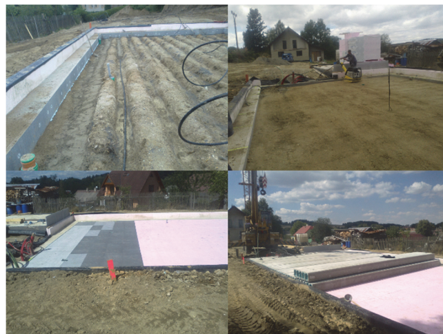
Figure 4 Realisation of a simple and a low-cost ground seasonal storage unit
