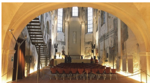
Figure 1 Interior of the church, after reconstruction
