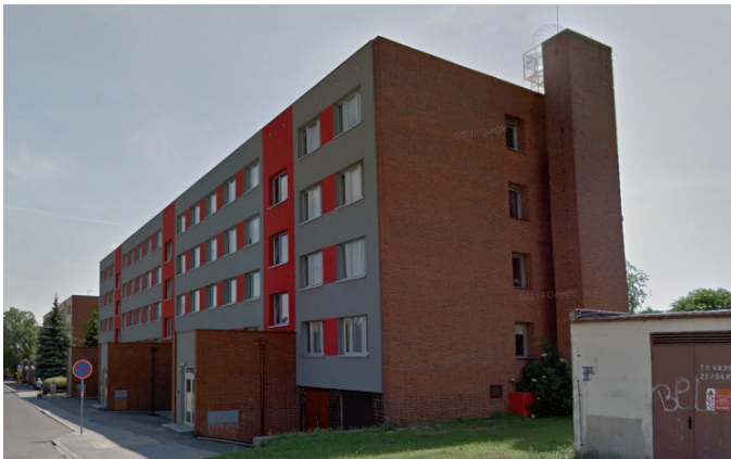
Fig. 2 Building 2 – the apartment block in Praha-Suchdol (source: www.mapy.cz)
