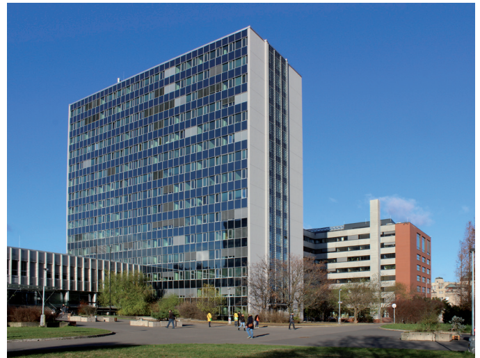
Fig. 3 Building 3 – Building A of the Faculty of Civil Engineering (source: cs.wikipedia.org)
