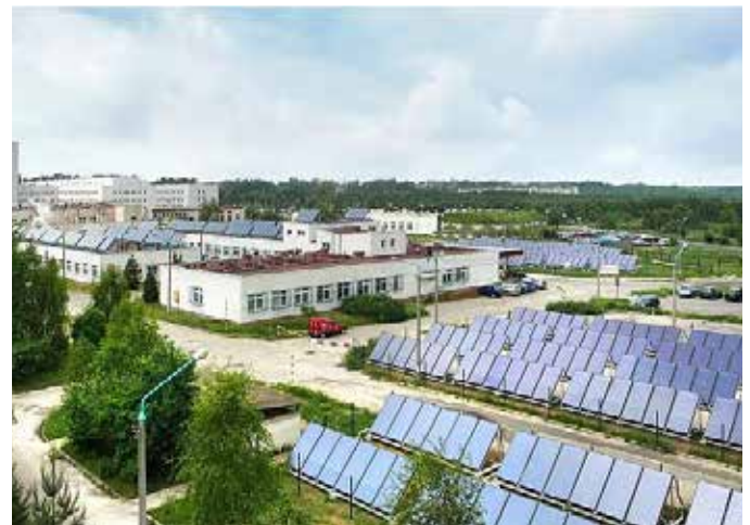
Figure 9 The solar panel system at the specialist hospital in Czestochowa (Viessmann)
