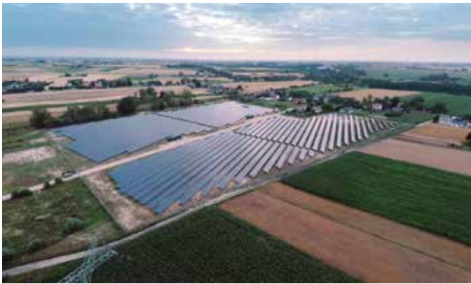
Figure 10 Czernikowo photovoltaic power plant (Energa)
