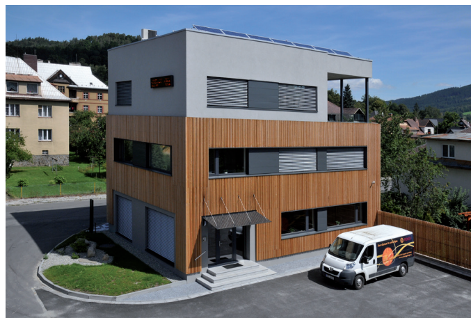
Obr. 1 Pohled na administrativní budovu Fig. 1 View of the administrative building
